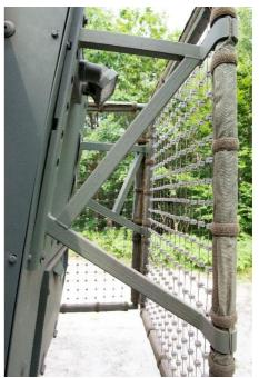
The individual net modules that form the protection system are connected with rigid screw joints or bands made of Velcro tapes. The net modules are mounted onto the object with adjustable brackets that set the distance between the net and the protected surface.
